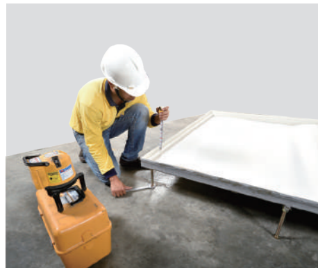
1. Floor base install
