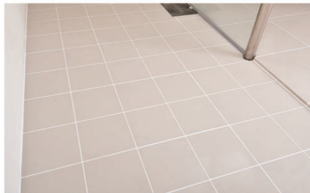
Small size tiles to create anti-slip function
