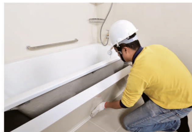
Removable side panel to have easier repair
